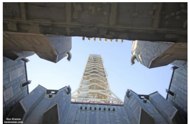
Looking up from beneath the enlarged exhaust hole of the Mobile Launcher to the 380 foot-tall tower astronauts will ascend as their gateway for missions to the Moon, Asteroids and Mars. The ML will support NASA's Space Launch System (SLS) and Orion spacecraft during Exploration Mission-1
