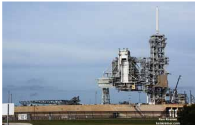
SpaceX transporter erector for Falcon rocket family rests atop ramp at Launch Complex Pad 39A at NASA’s Kennedy Space Center in Florida. It will transport and erect SpaceX Falcon 9 and Falcon Heavy rockets between processing hangar and launch pad. It was to be used for upcoming hold down static fire test of recently recovered Falcon 9 booster. Formerly served as NASA space shuttle launch pad 39A. Credit: Ken Kremer/Kenkremer.com
